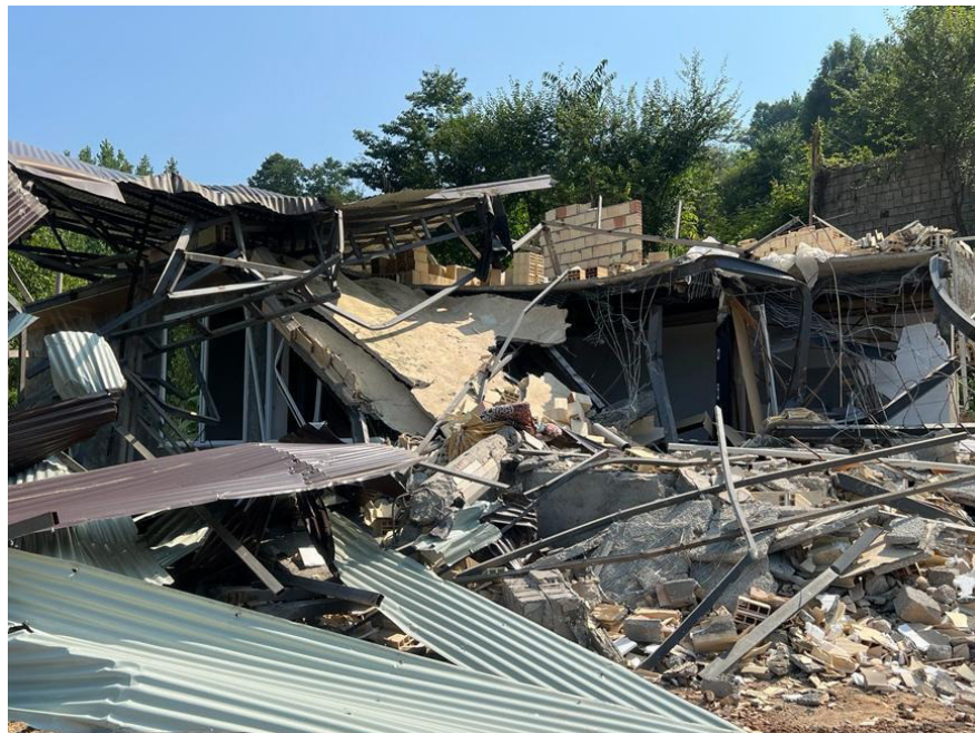
Destroyed Bahá'í homes (Credit: Bahá'í International Community)
